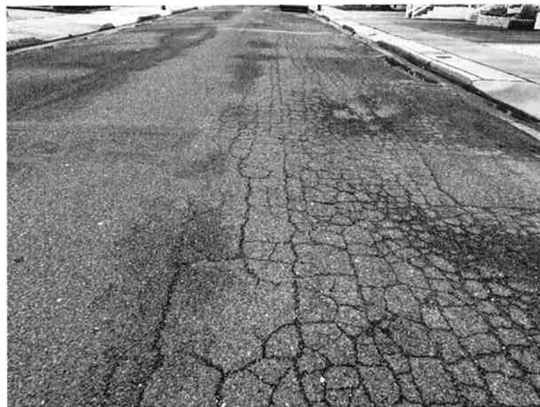
Photo 4 – Multiple cracking
