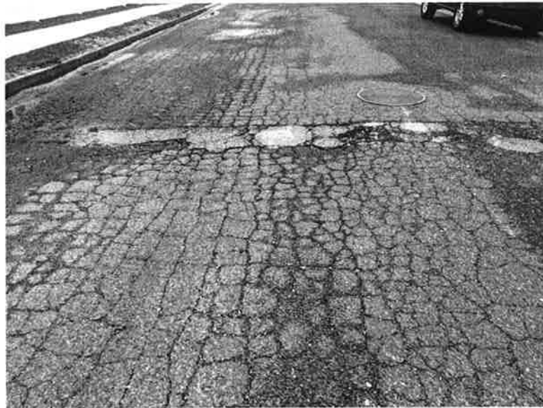
Photo 3 – Multiple cracking
